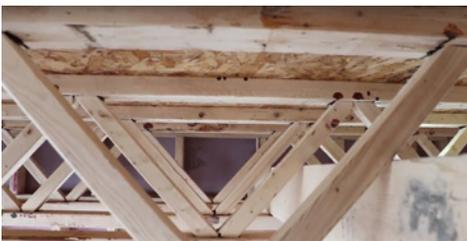
2x6 strongbacks are attached perpendicular to the joists to increase transversal rigidity of the floor system. Tying the joists together with strongbacks enables the floor system to react to vibration as a cohesive unit. Strongbacks are a simple and economical solution offering floor performance that's greatly appreciated by customers.
